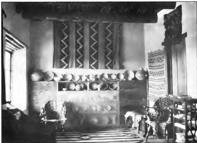
Figure 4.2. The Morris living room with collections of Indian objects. Ceiling beams are twelfth-century elements removed from the West Ruin. Window and door lintels are modern wood installed in the Anasazi way.
